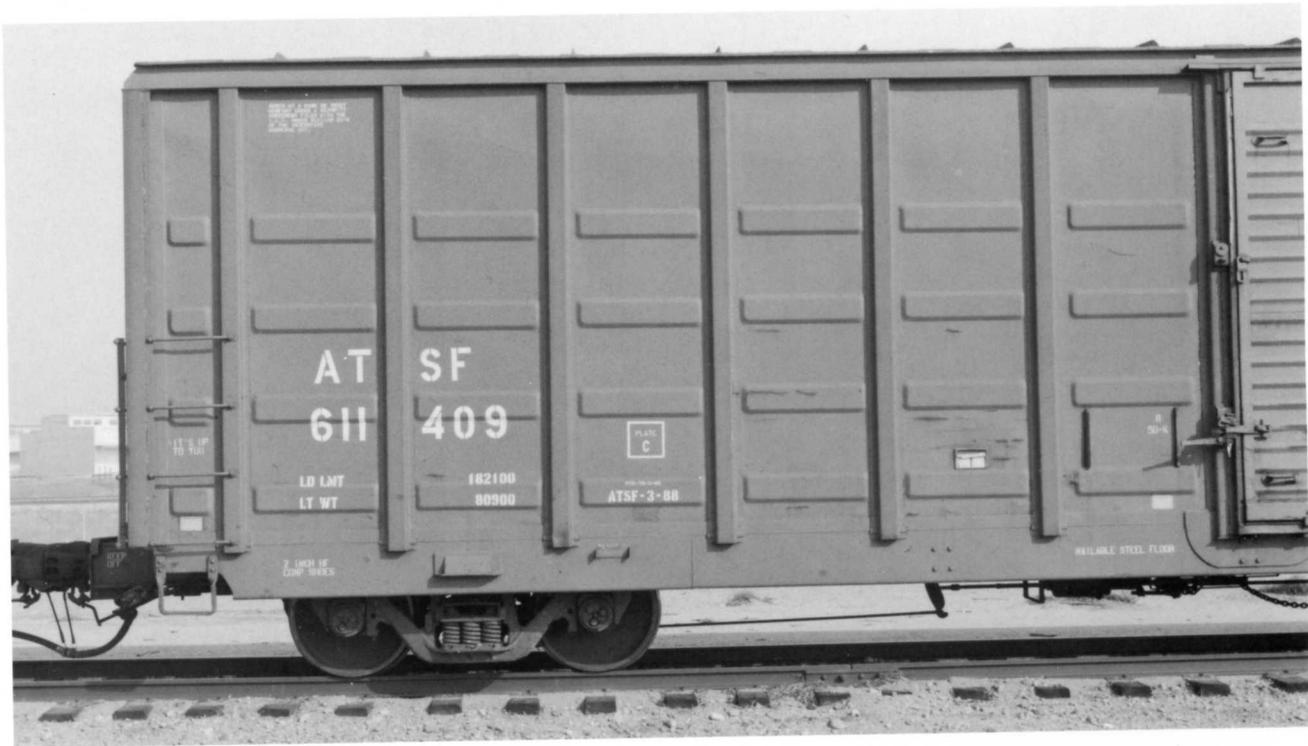
**ATSF 611409** (Above). Left side detail. The cars are equipped with nailable steel floor. Notice how the four rows of waffles are placed toward the bottom of the sides.
