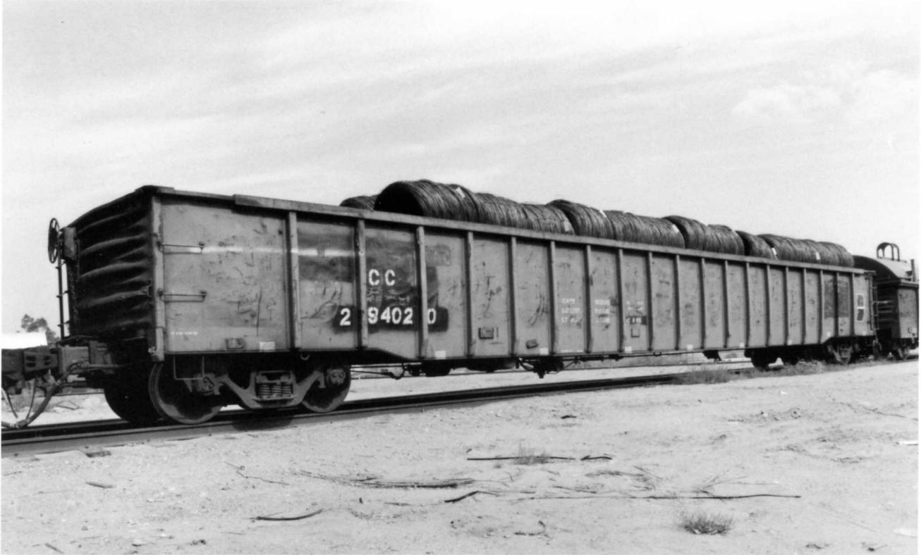
**CC 294020** (Above) is the last car of the CC 294001-294020 series. The car has a 65'6" IL. Inside height is 5'0". Inside width is 8'11". Note the top reinforcement angle and nineteen side posts. The middle 15 side posts are tapered at the bottom. The outer two side posts on each end have squared bottoms. All welded design.
