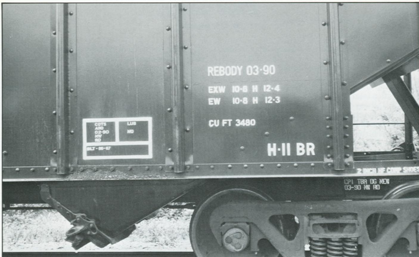
NW 3696. Detail of "A" end side showing rebody stenciling, cuft capacity, dimensions, new class, and consolidated stencil.
