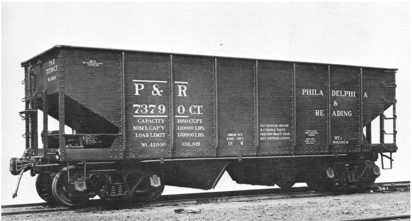
P&R 73790, class HTJ was built 8-12-19 by the Ralston Steel Car Co. at Columbus, Ohio. Note the cubic capacity is the same (1880 cuft) as the Standard Steel built P&R 77004.
