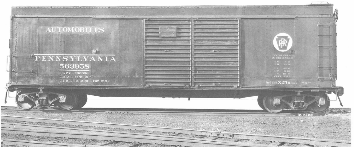
Pennsylvania RR 563958, X25B was an experimental attempt to increase the headroom in the X25A, three such cars were rebuilt, plus a fourth X25C which tried to meet the same goal with a PRR round roof replacement. Government financing for large numbers of new roundroof box and auto box cars probably had something to do with the decision to not pursue this work. Richard Burg Collection
